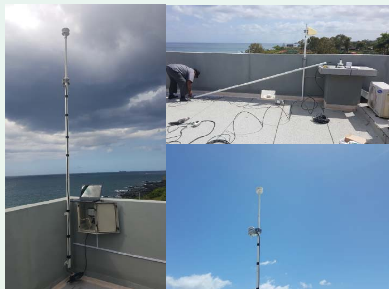
Figure 3 - Installation of weather station at the MOI.
